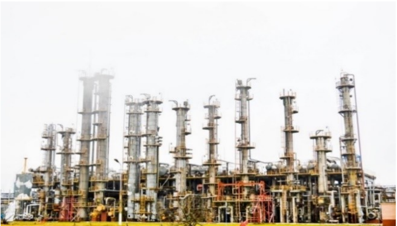
Figure 1. Air Separation Unit (Bolbik 2017)
